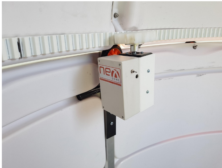
Figure 3: Motor unit mounted.
